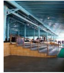
Figure 46. Corridor in Surakarta Great Mosque
