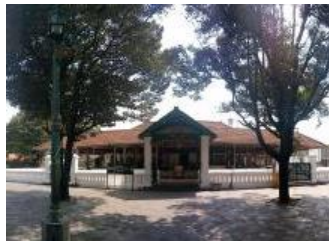
Figure 13. Courtyard of Kotagede mosque
