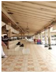
Figure 44. Corridor in Yogyakarta Great Mosque
