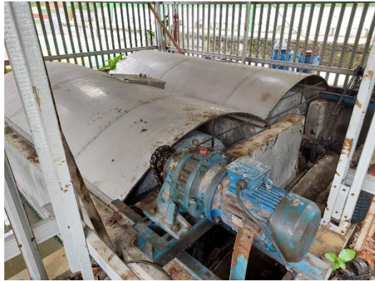
Gambar 4. 3 Unit pengolahan rotating biological contactor
