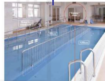
(9) A warming room is installed so that children who have difficulty in temperature control can use the swimming pool safely. The water depth is set at three levels (gangs for wheelchair, 60cm depth and 1.20m depth) considering use in wheelchairs and the physical sizes of children.
