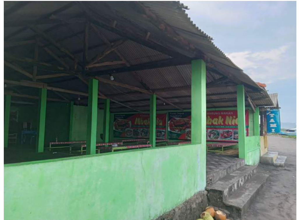
Figure 2.10: Site Condition Source: Author
