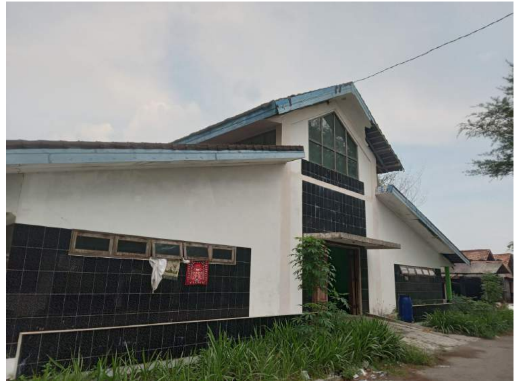
Figure 2.5: Site Condition Source: Author
