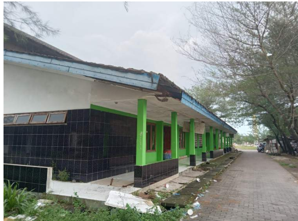
Figure 2.7: Site Condition Source: Author
