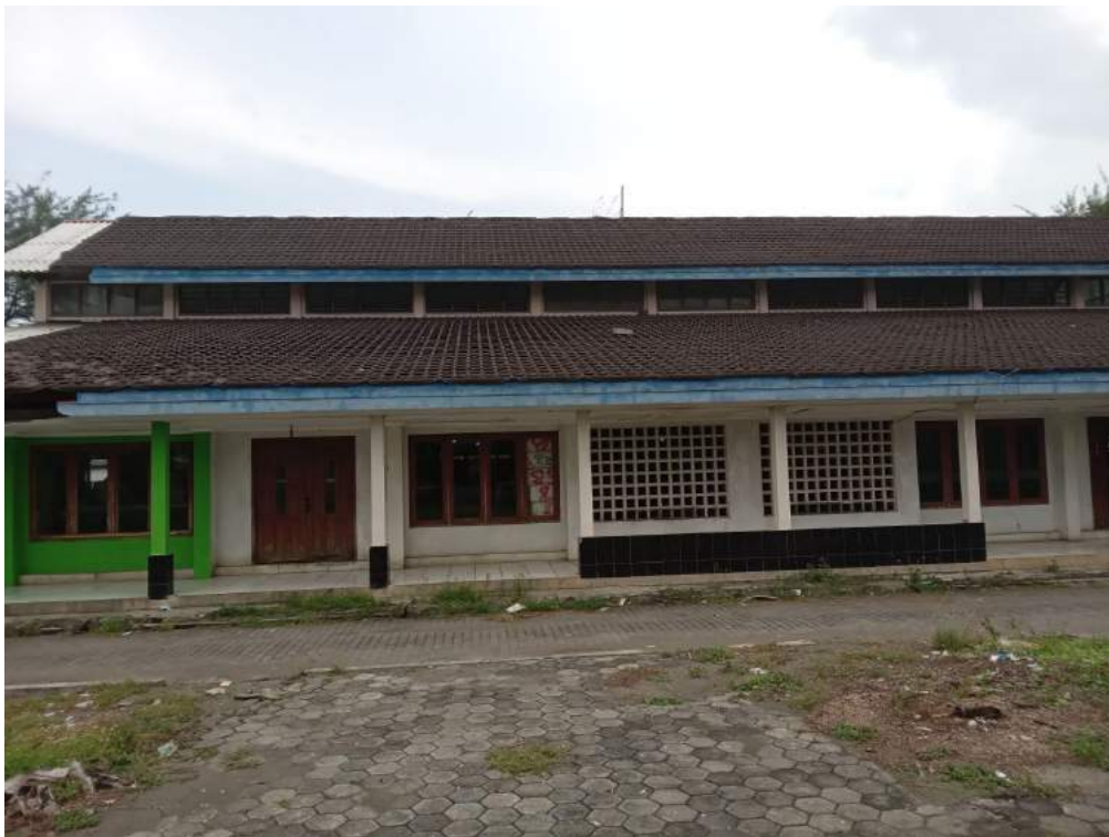
Figure 2.6: Site Condition Source: Author
