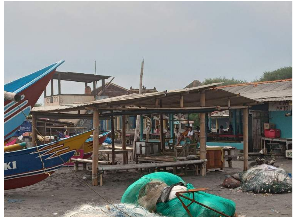
Figure 2.12: Site Condition Source: Author
