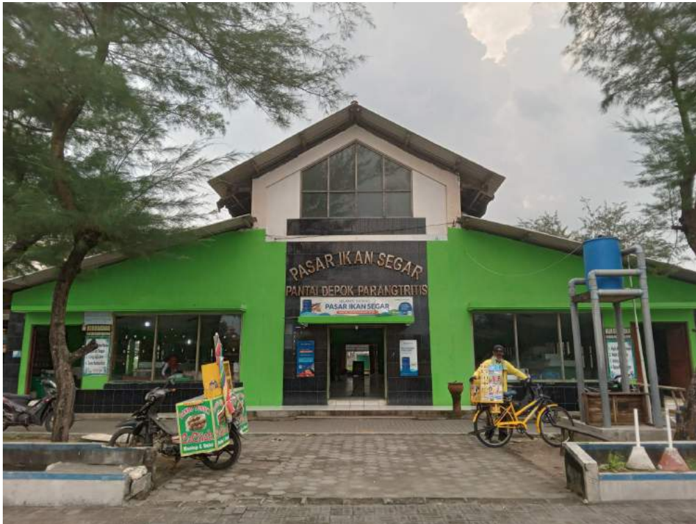
Figure 2.4: Site Condition Source: Author
