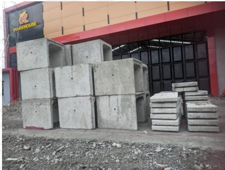
**Gambar L 3.2 Beton *U-ditch Precast* Sebelum Dipasang Pada Galian**
