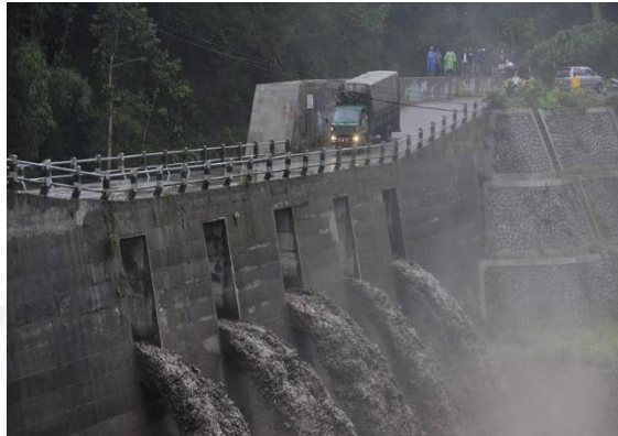
Gambar 3.7 Sabo Dam Tipe Tertutup
