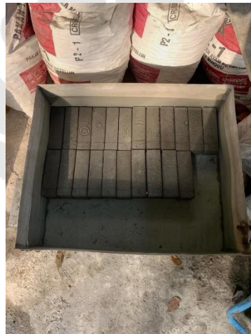
Gambar 4.18 Proses Perawatan Paving Block
