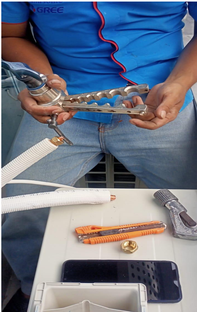
Gambar L-3.3 Proses Blering Pipa Refrigerant
