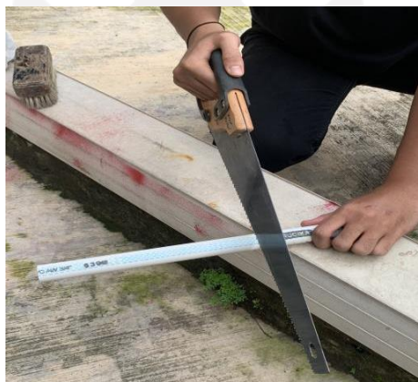
Gambar 4 - 1 Pemotongan Pipa 3/4 Inch.
