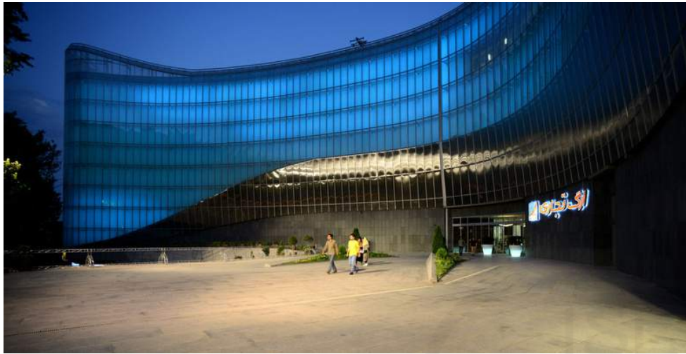
Gambar 2.46. Fasad ARG Shopping Mall Sumber: archdaily.com
