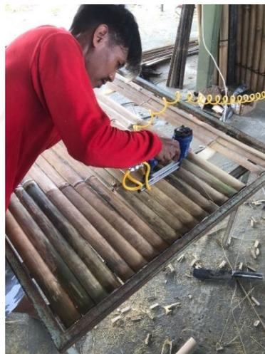
Gambar 4. 6 Proses Staples Bambu
