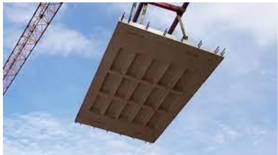
**Gambar 3.4** Beton Pracetak Flyslab
