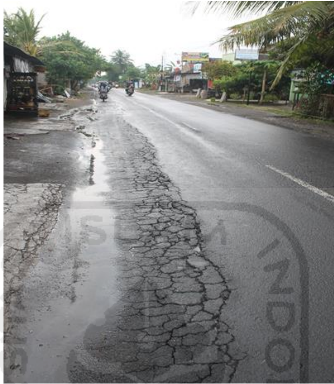
Gambar 2-4 Alligator Cracking
