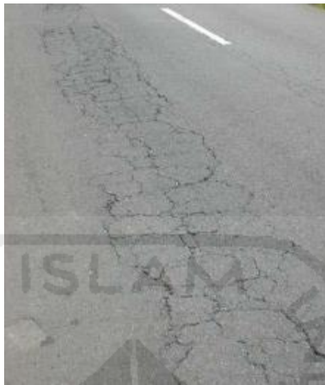
Gambar 2-1 Block Cracking
