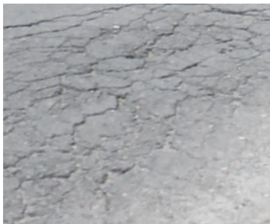
Gambar 2-3 Alligator Cracking
