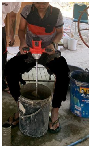
Gambar L-1.7 Proses Mixing Adonan Bata Ringan
