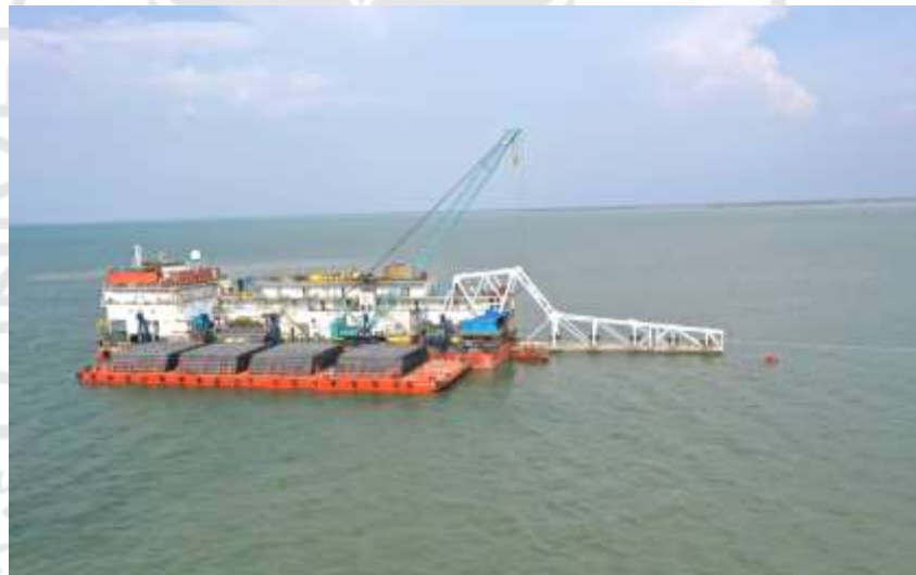
Gambar 5.7 Instalasi Subsea Pipeline
