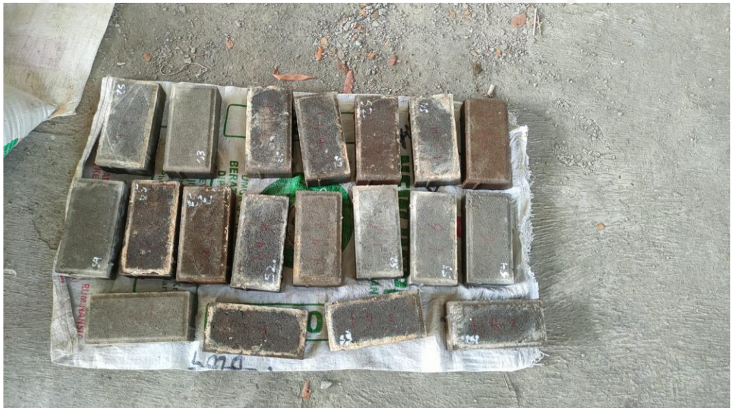
Figure 5.2 Reddish Looking Paving Blocks due to Corrosion
