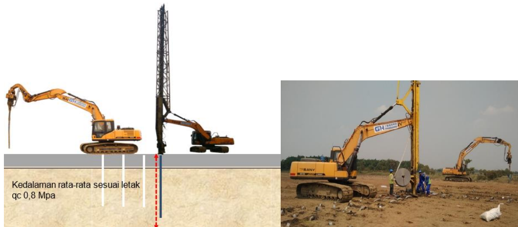
Figure 3.14 Installation of PVD
