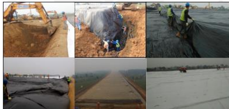
Figure 3.18 Sealing Ditch Installation
