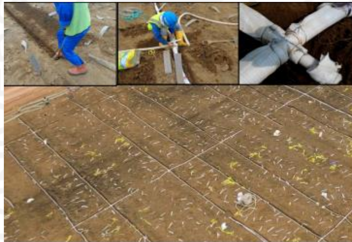
Figure 3.16 Installation of PHD
