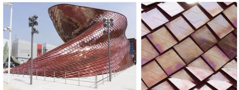
Gambar 2.19 Photocatalytic Ceramic Self-cleaning Facade
