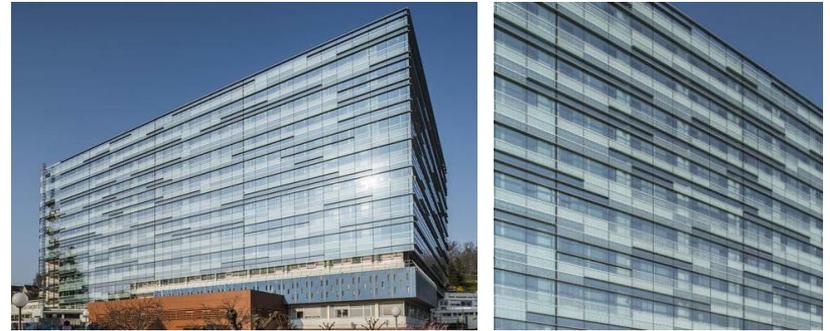
Gambar 2.18 Photocatalytic Glass Self-cleaning Facade
