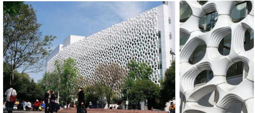
Gambar 2.22 Photocatalytic Concrete Self-cleaning Facade
