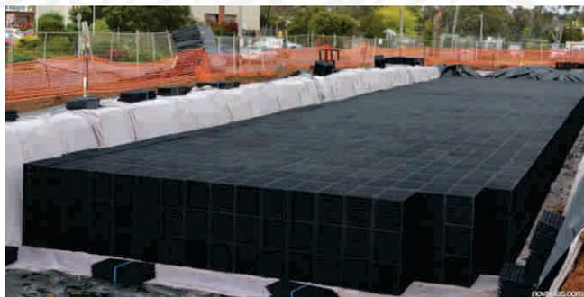
Gambar 3.3 Stormwater Module
