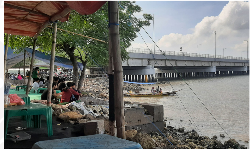
Figure 54. Site Condition Documentation Source: Author, 2022
