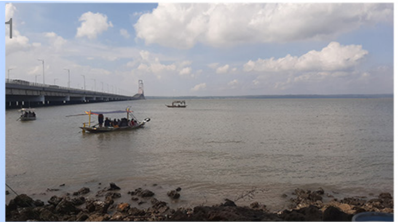
Figure 47. South-Front View Source: Author, 2022
