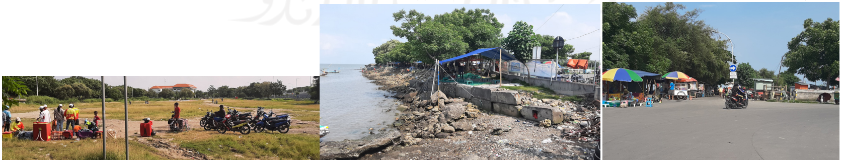
Figure 56. Site Condition Documentation Source: Author, 2022
