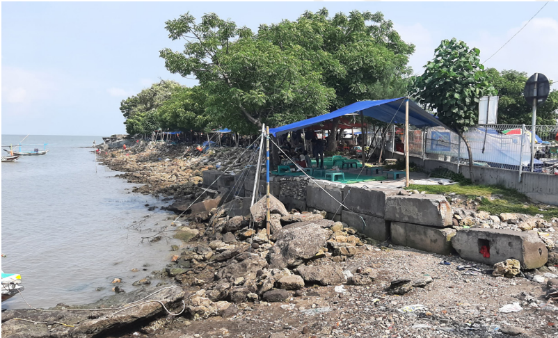
Figure 53. Site Condition Documentation Source: Author, 2022
