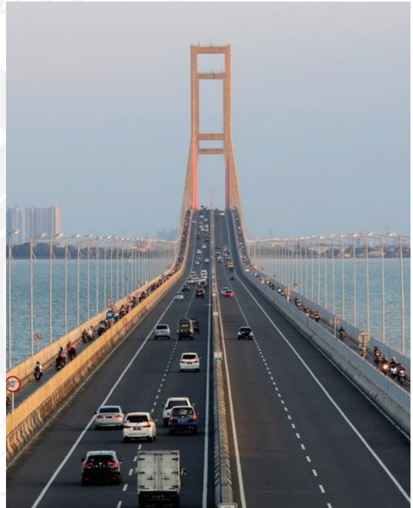
Figure 15. Suramadu Bridge Source: https://investor.id/
