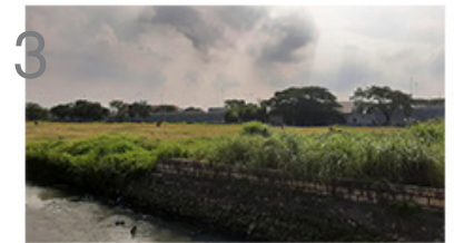
Figure 49. West View Source: Author, 2022
