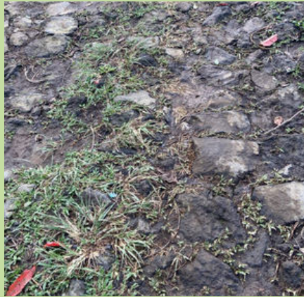
The site road texture
