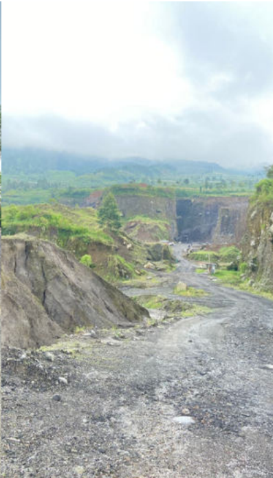
Enter site location
