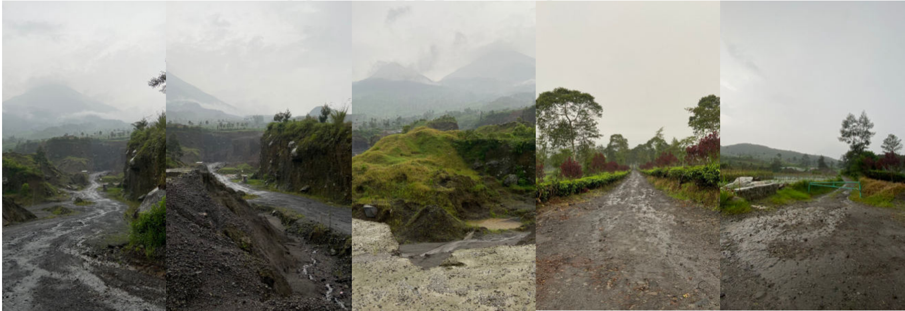
Access on the site
