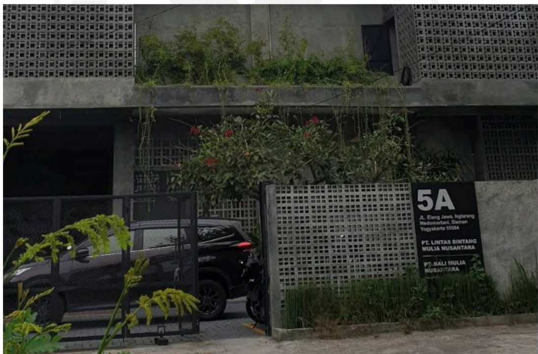
Figure 4. 2 Starcross Headquarter (SH) Building
