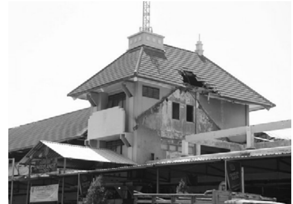
Figure 1.2 Public Building, Pasar Legi Ponorogo Source : Author, 2021
