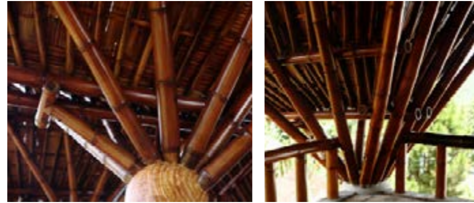
Figure 2.38 Structure Detail, Chicken Comb Source : Archdaily.com, 2021
