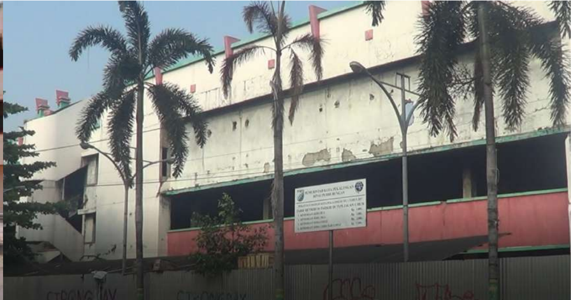
Picture 1.4 Borobudur Mall building Source: Batik TV, 2020
