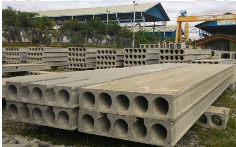
Gambar 3.5 Precast Full Slab di Stockyard
