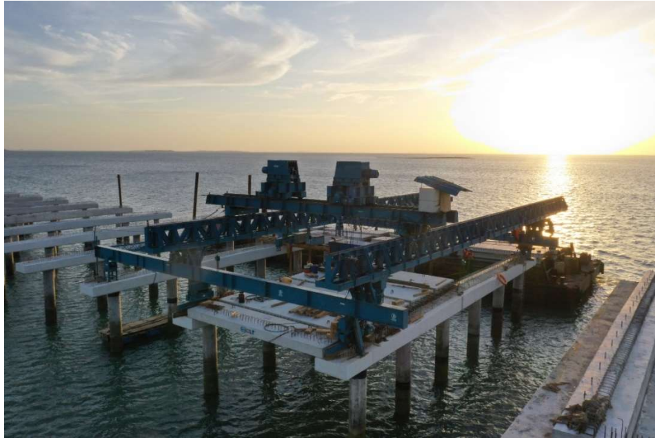
Gambar L-1.1 Launching Gantry
