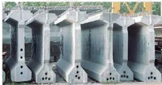
Gambar 3.5 Balok Girder Tipe PC-I
