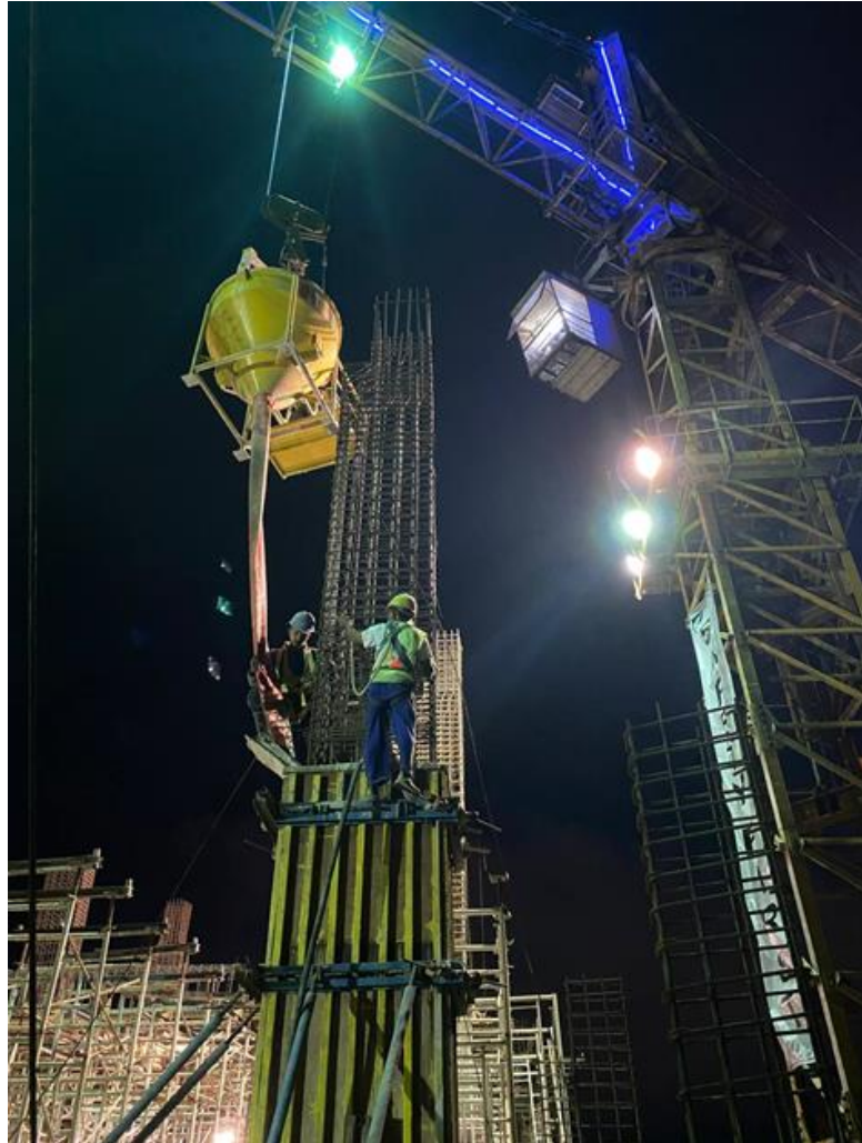
Lampiran 4.15 Gambar Pengcoran Concrete Bucket
