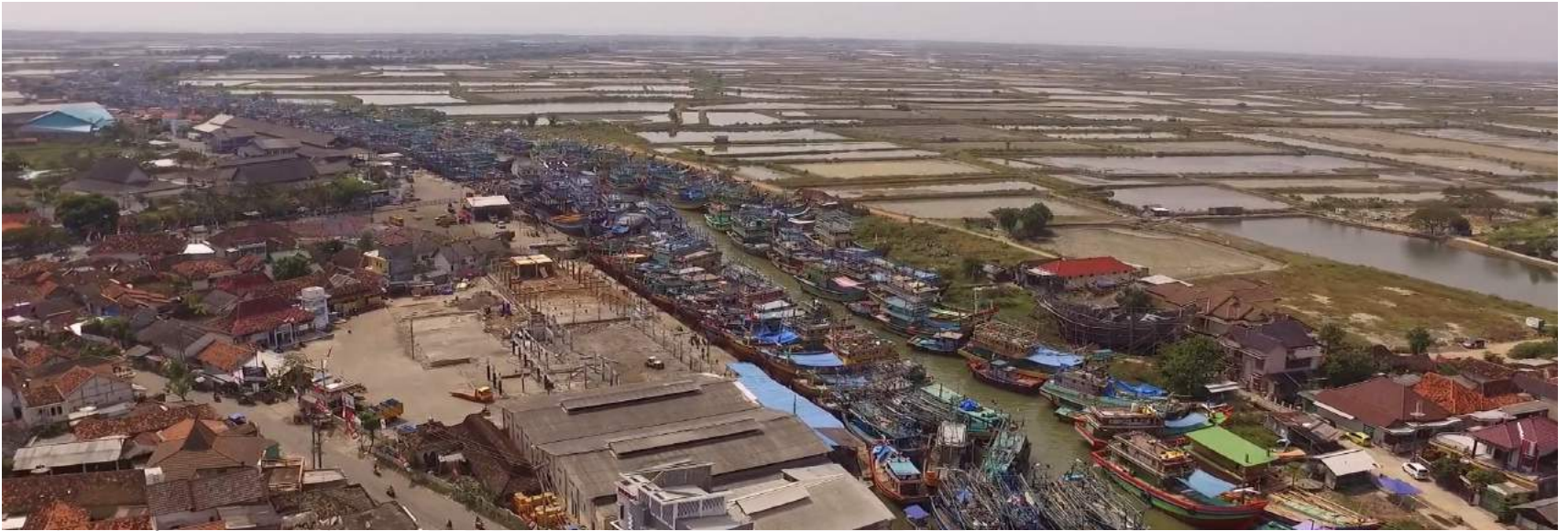
Aerial Picture of TPI Juwana I and TPI Juwana II
