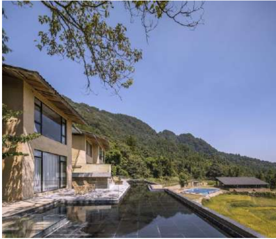
Gambar 2.60 Dianjing Bagu Suji Hotel Sumber : Arch Daily, 2021
