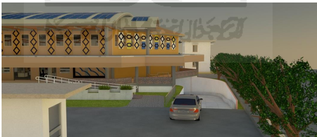
Gambar 4.1 15. Entrance Ramp parkir motor & mobil.
