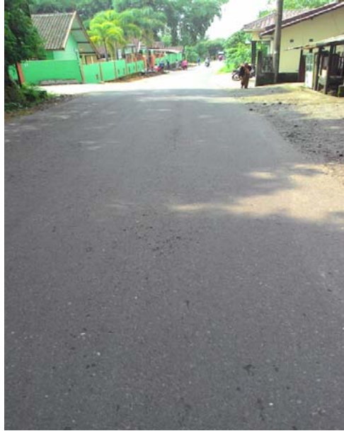
Gambar 5.1 kondisi jalan rating good
