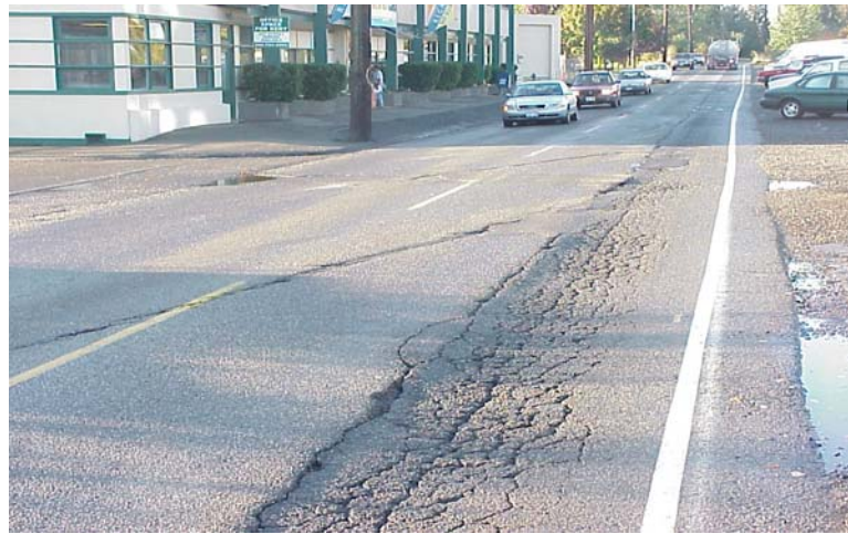
Gambar 3.5 Alur ( Rutting )
