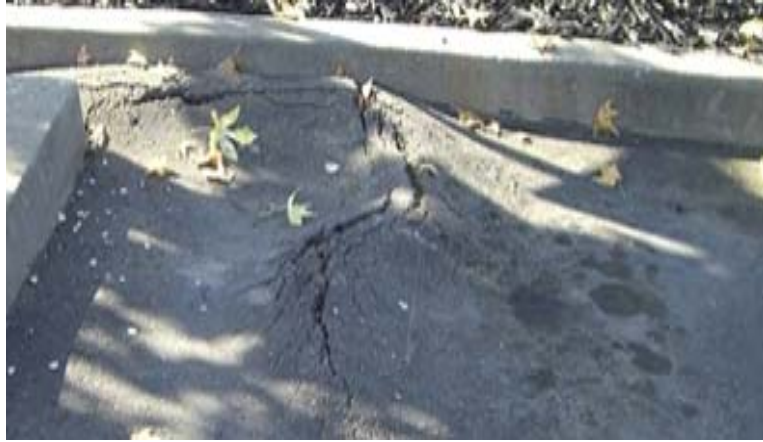
Gambar 3.8 Jembul ( Upheaval )
