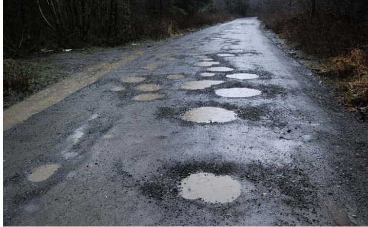
Gambar 3.9 Lubang ( Potholes )
