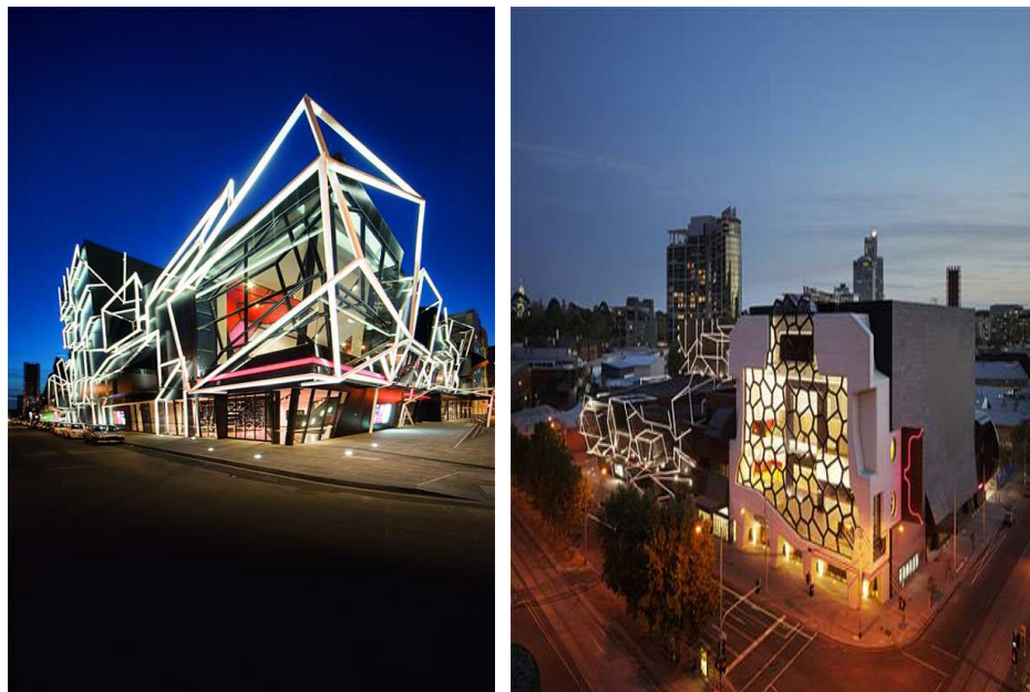
Gbr.2.18 Modern Theater Building in Melbourne Sumber: www.designshoot.com
