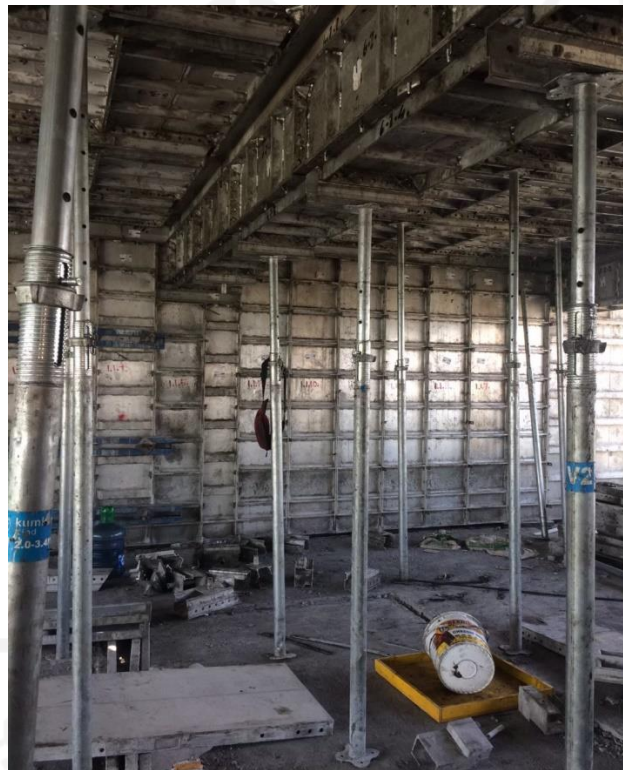
Gambar 3. 2 Bekisting aluminium
