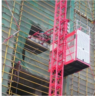
Gambar 3.16 Material Hoist
