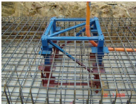
Gambar 3.11 Pondasi Tower Crane
