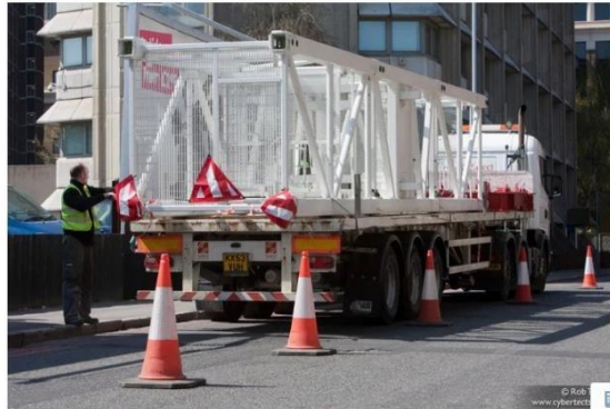
Gambar 3.13 Mobilisasi Segmen Tower Crane
