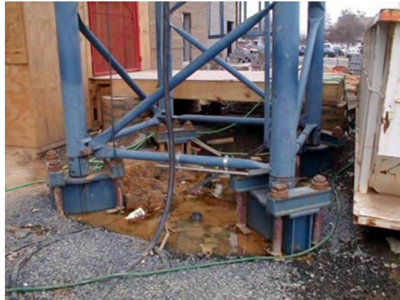
Gambar 3.12 Base Section dan Fine Angle
