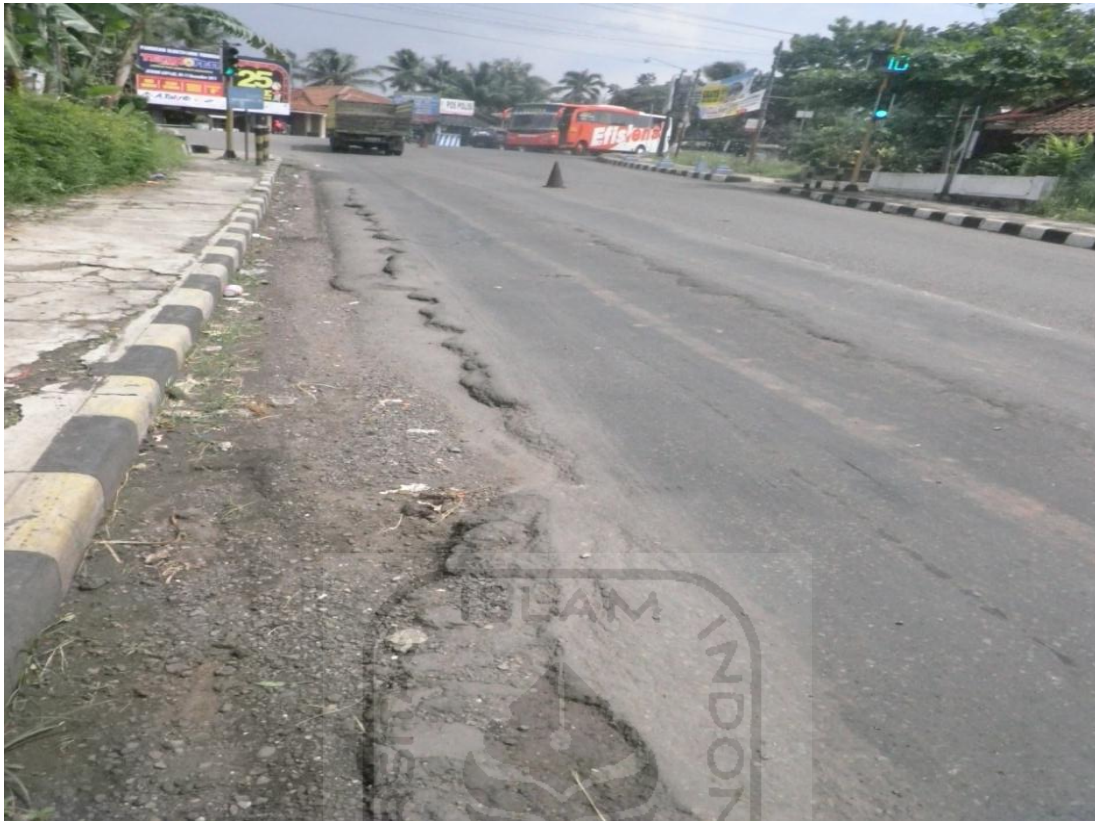
Gambar 5. Alur ( Rutting )
