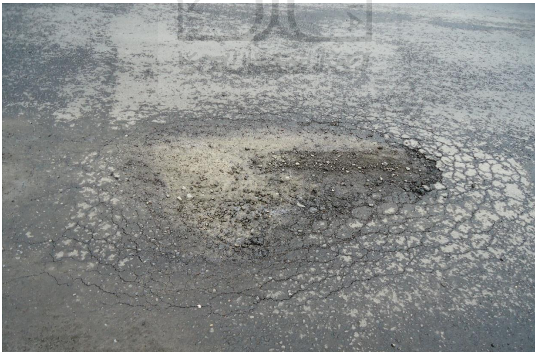
Gambar 6. Lubang ( Potholes )
