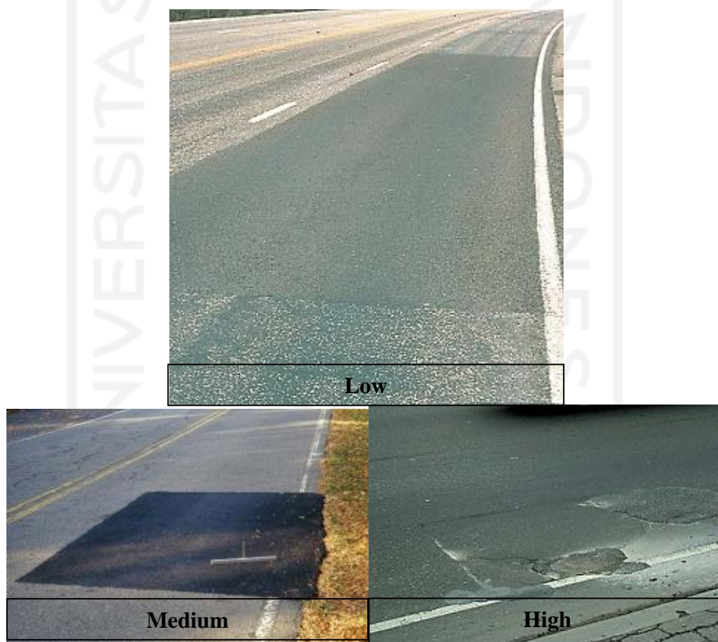
Gambar 3.15 Tambalan dan Tambalan Galian Utilitas ( Patching and Utility Cut Patching )
