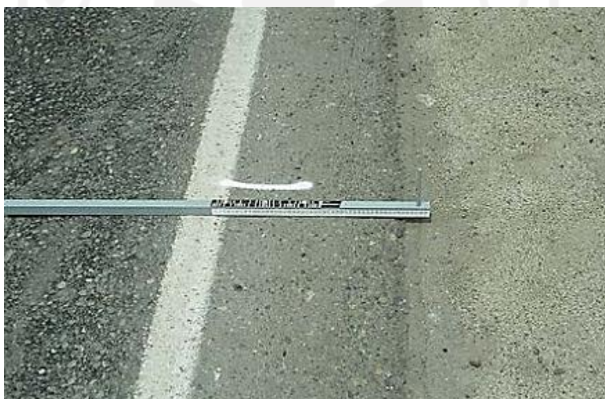
Gambar 3.11 Jalur/Bahu Turun ( Lane/Shoulder Dropp-Off )
