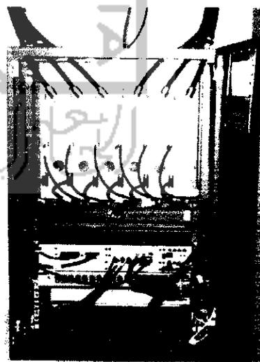
**Gambar 4.9 *BTS* Huawei Unit Indoor 3900**
