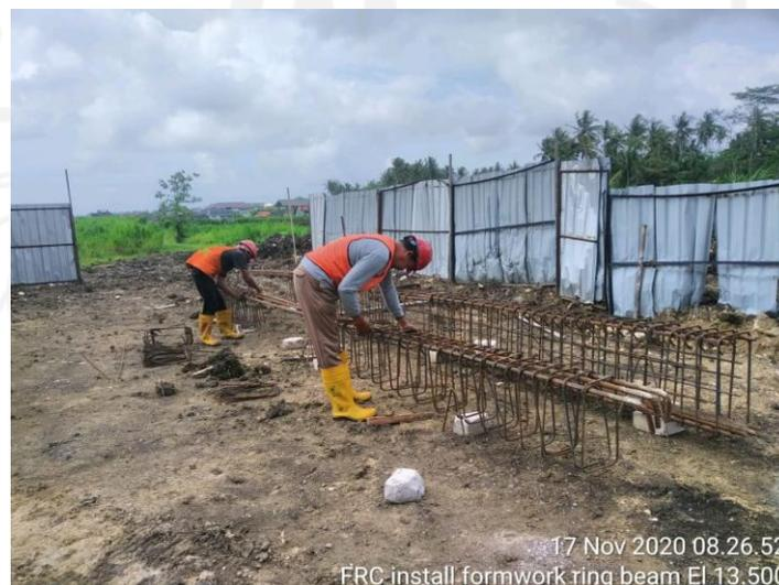
**Gambar 5.14 Proses Pembesian Ring Beam**
