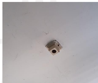
Gambar 5.27 Fitting tanpa Bohlam Lampu
