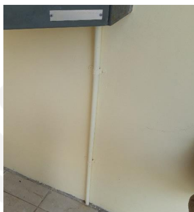
Gambar 5.29 Grounding Listrik
