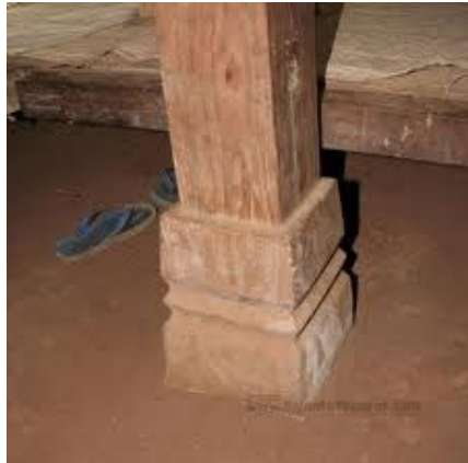
Gambar 2.17 Pondasi Umpak
