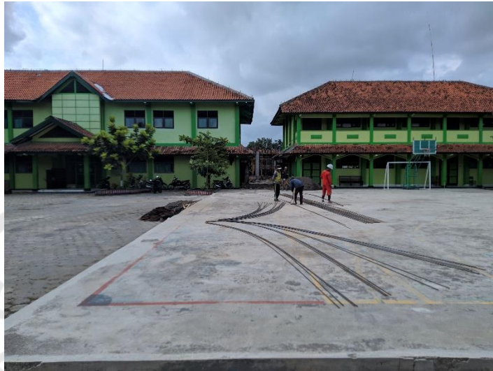
Gambar L-2. 9 Unloading Area Besi
