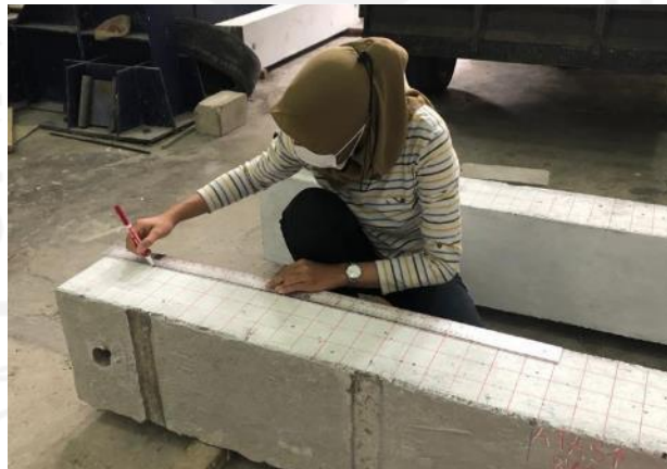
GAMBAR 28 MARKING BALOK BETON
