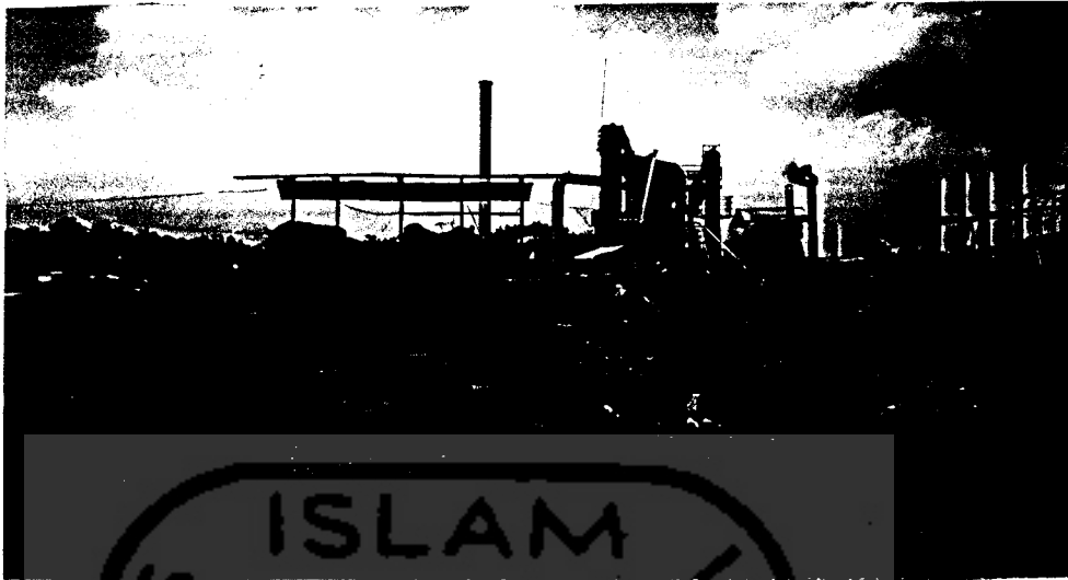
Gambar 3.8. Asphalt Mixing Plant di Base Camp
