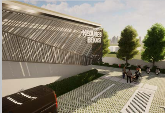
Application of secondary skin on the first building mass
