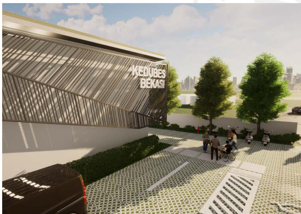
Application of secondary skin on the first building mass
