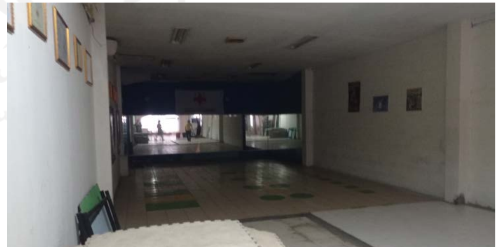
Figure 2.14 Existing condition of Multifunction room Source : Author
