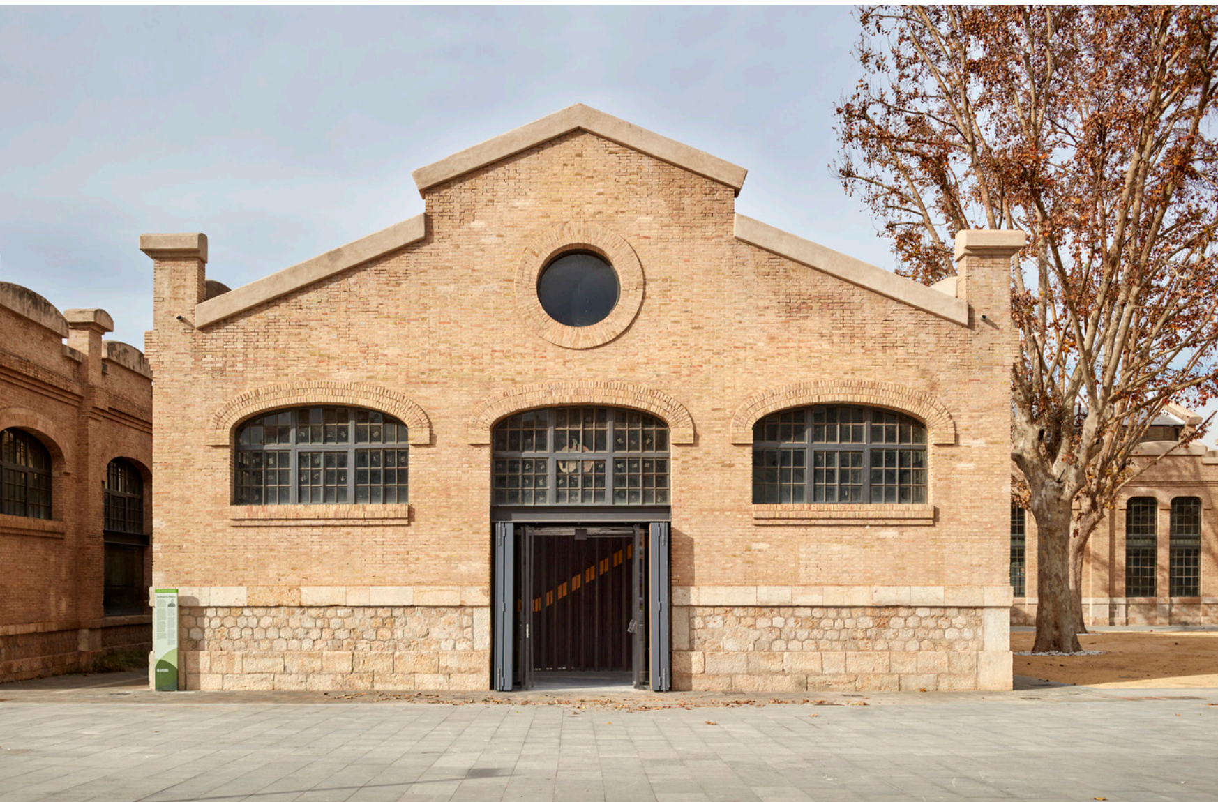
Figure 2.30 Hall 3 of the Parc Central
