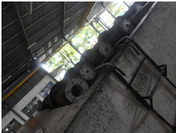
Gambar 4.7 Bak penampungan poses steam
