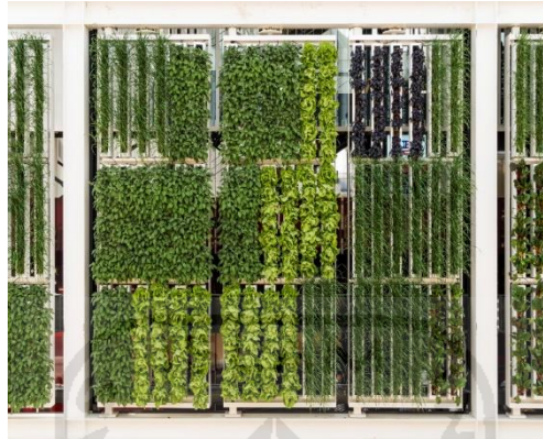
Gambar 2.46 Fasaad USA Pavillion - Expo Milano 2015
