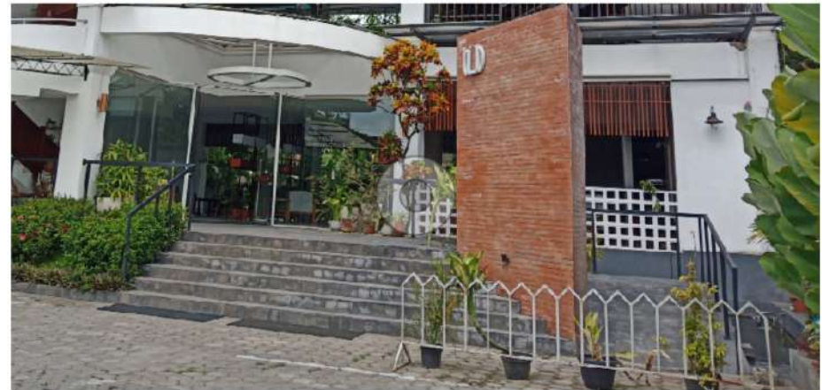
Gambar 4.32 : Entrance Existing Hotel Sumber : Penulis (2019)
