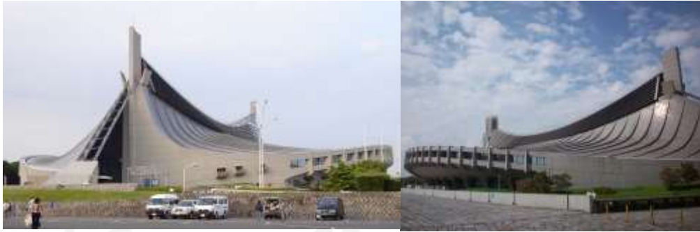
Gambar II. 52 : Tampak Yoyogi National Gymnasium
