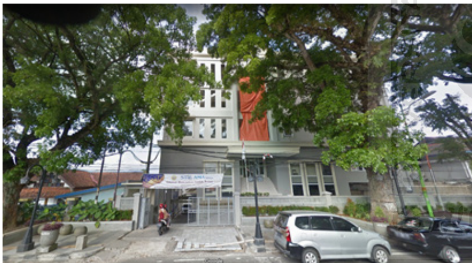
Figure 2.11 South East Boundary (source: Author, 2021)
