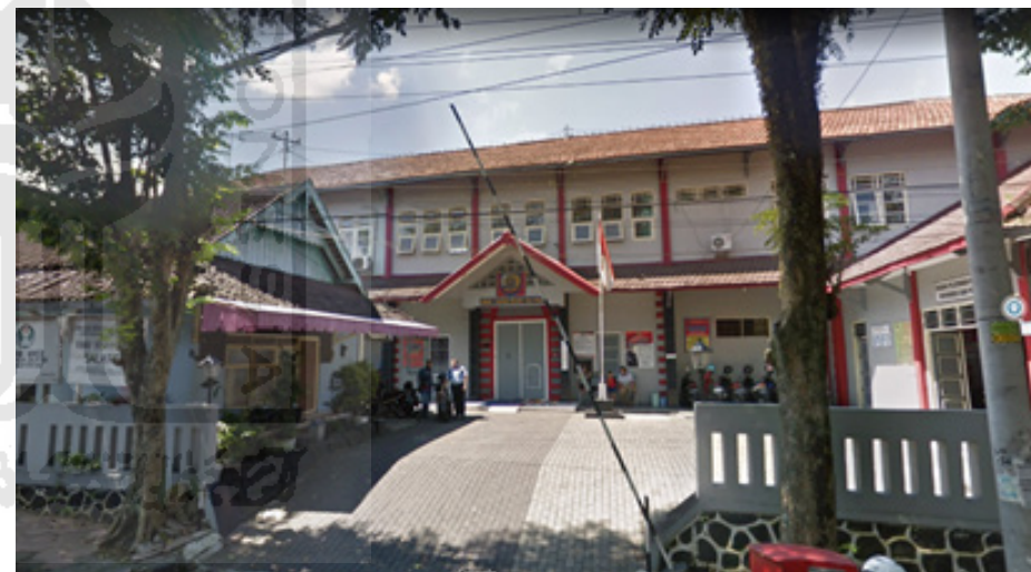
Figure 2.13 South East Boundary (source: Author, 2021)
